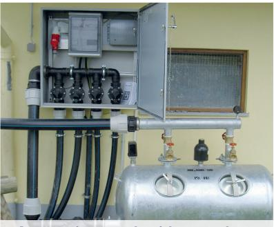
Automatic controls with manual filter system
